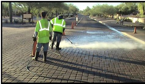
The Clean Water Act requires full reclamation and the waste water generated from the high pressure washing process to be thoroughly filtered, and all solids, fines and Class II hazardous materials (petroleum products) to be safely and effectively removed and separated from the
